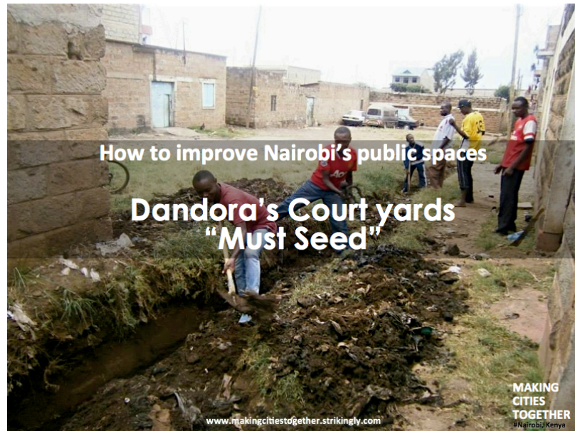
Figure 1 "Must Seed" - Rehabilitation work of one of Dandora Courtyards[]
