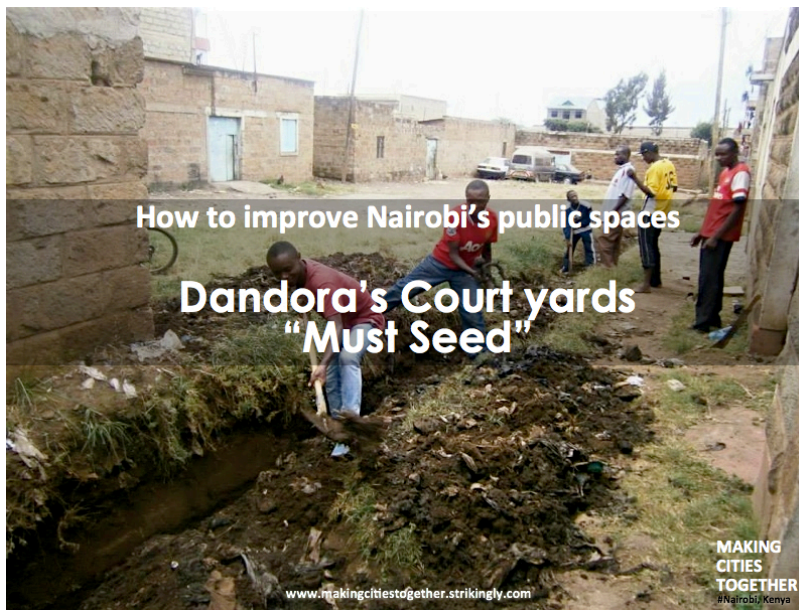
Figure 1 "Must Seed" - [ ]Rehabilitation work of one of Dandora Courtyards
